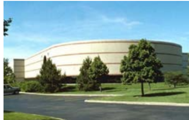
Pictured: Hanna Cylinders has signed a long-term lease to occupy 105,637-square-foot facility at 8901 102nd Street in Pleasant Prairie.
